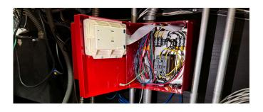
The IQ2 Smart Controller provides an effective way to remotely diagnose STP alarms.
